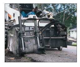
The **oscillation** of the planer is free to rotate, providing optimum surface tracking and isolating the planer from loader movements caused by uneven terrain. Adjustable depth skis allow tapering of cut, such as when matching two uneven pavement surfaces or removing a curb ridge. (Not available on 15-in. curb planer.)
