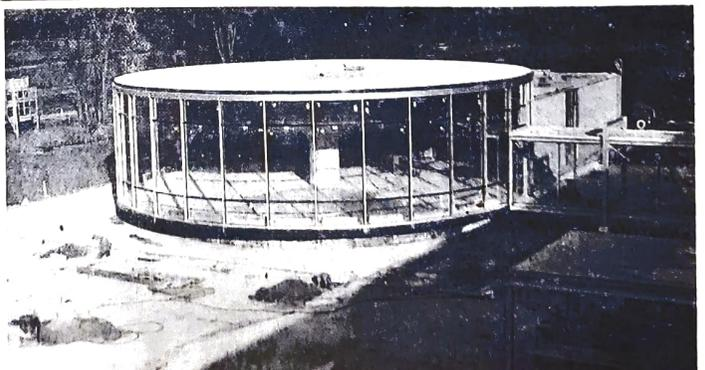
Striking design of the cafeteria forming part of CIDA Company Limited's new plant on Metropolitan Boulevard shows the mushroom-pillar and the plate-glass panels during construction. The cafeteria stands in an artificial pond and is connected to the general offices by a glassed-in walkway. Operations at the new plant are scheduled to start Nov. 23. Henry Kara Photo
