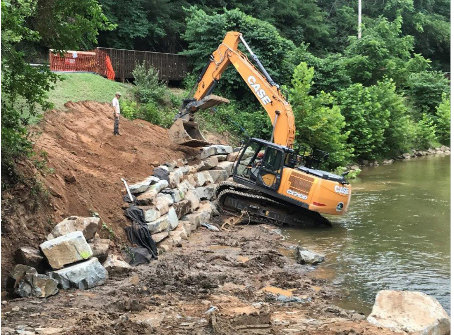
FORVA is restoring a riverbank on the Pigg River in Franklin County. Part of developing a new Franklin County Blueway
