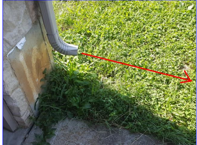
2.3 Item 2(Picture) rear right corner of home
