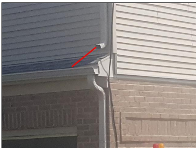
2.3 Item 6(Picture) rear right corner of home
