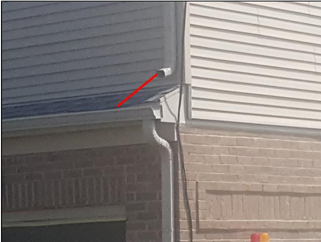
2.3 Item 6(Picture) rear right corner of home
