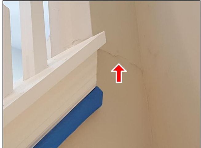
6.1 Item 2(Picture) top of staircase
