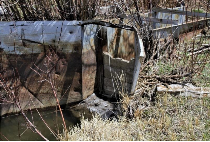
Headgate looking downstream
