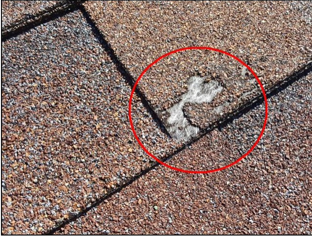
2.0 Item 1(Picture) below master bedroom area rear of home
