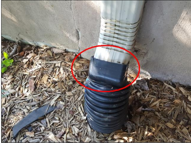
2.3 Item 7(Picture) front left corner of home
