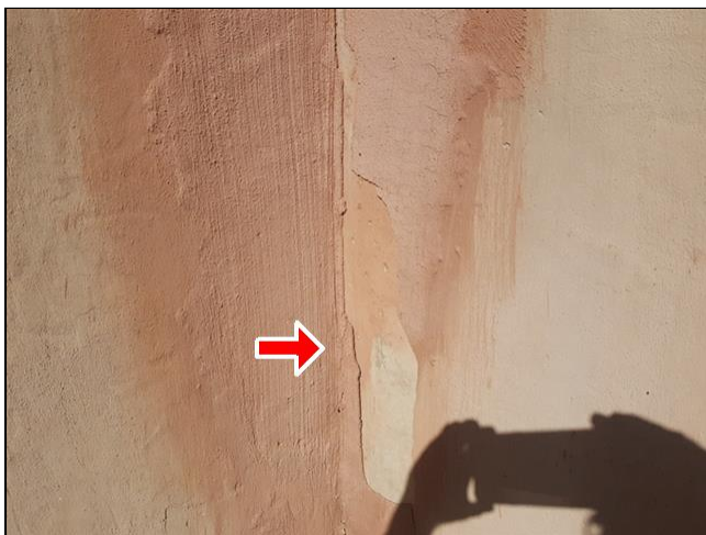
1.1 Item 12(Picture) rear right corner of home
