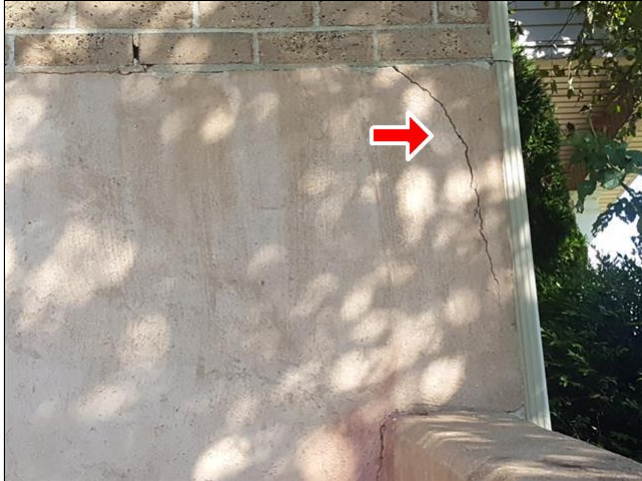
1.1 Item 10(Picture) front left corner of home
