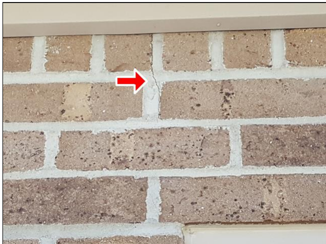
3.0 Item 2(Picture) above garage left corner
