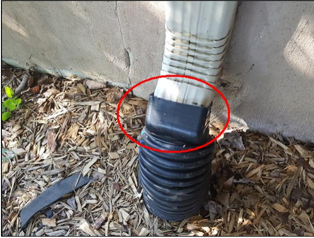
2.3 Item 7(Picture) front left corner of home
