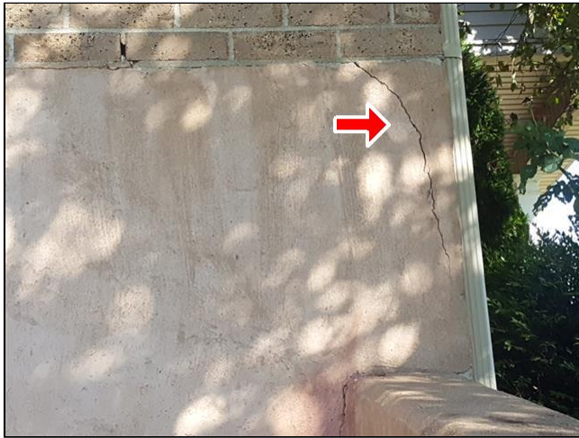
1.1 Item 10(Picture) front left corner of home
