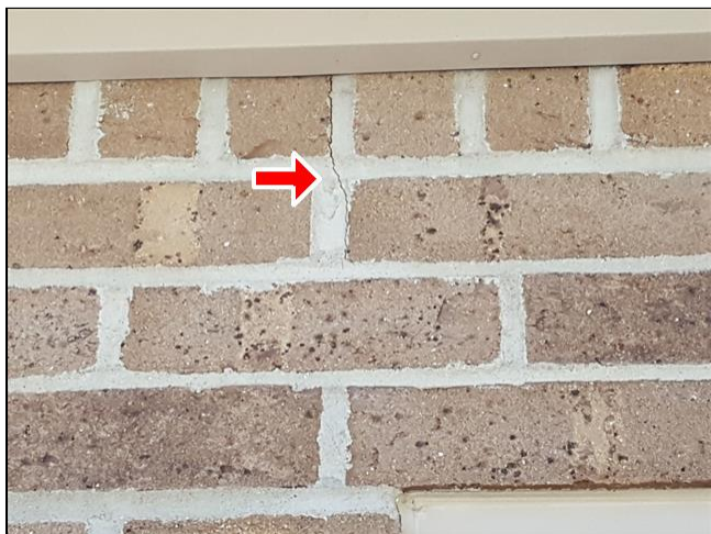
3.0 Item 2(Picture) above garage left corner
