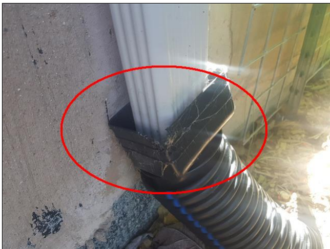
2.3 Item 11(Picture) rear right corner of home
