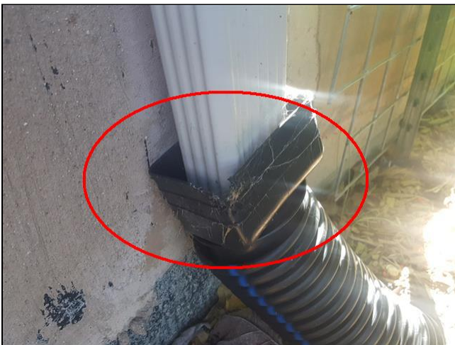
2.3 Item 11(Picture) rear right corner of home
