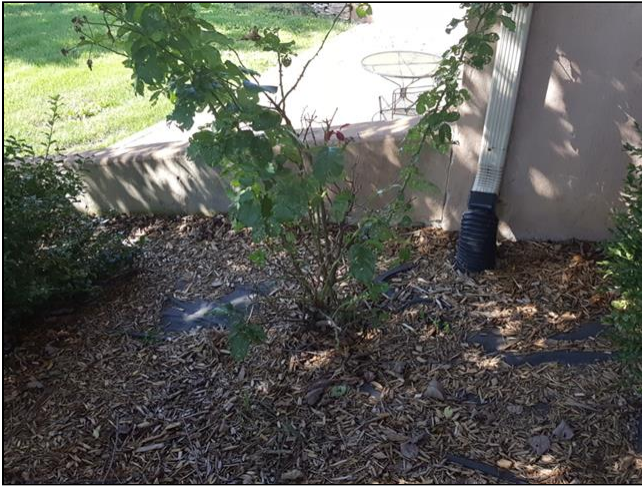
2.3 Item 1(Picture) front left corner of home
