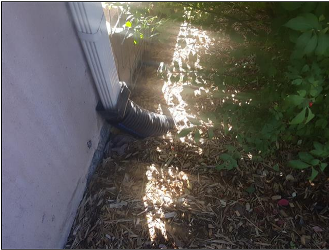
2.3 Item 3(Picture) rear right corner of home
