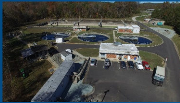
Roxboro treatment plant
