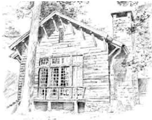
Camp Uncas Dining Room Building, Window with true divided lights.
