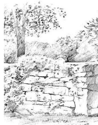
Dry stacked stone retaining wall
