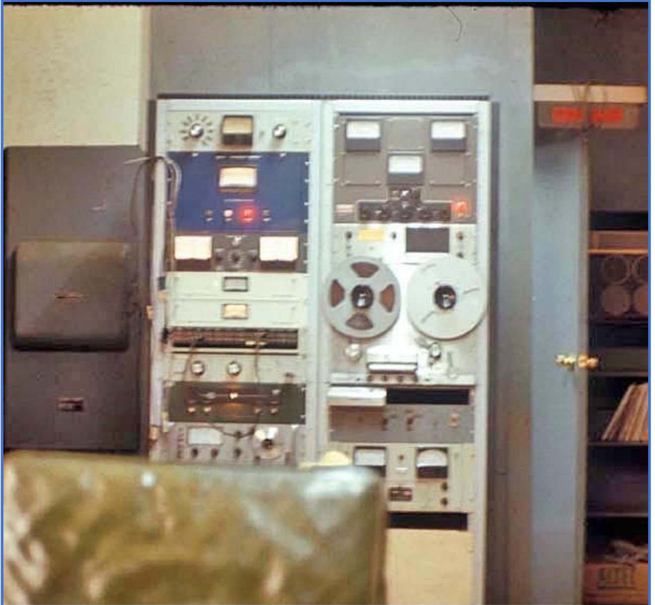
These are the tape recorders in the AM radio station. You can see the red "ON AIR" sign and door to the control room on the right.
