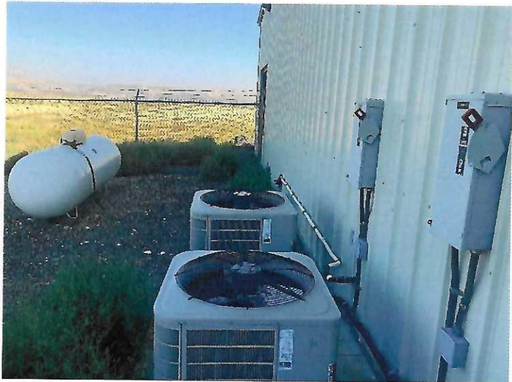
View along W side of building
