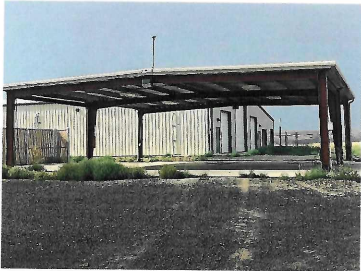
View facing N from fenced entry gate
