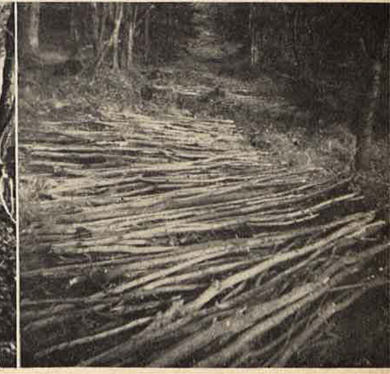
WE BUILT CORDUROY ROADS ACROSS SWAMPS. NO VERY SMOOTH, BUT KEPT US FROM MIRING.
