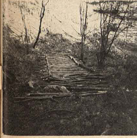
WE CUT POLES AND BUILT BRIDGES. THIS ONE IS A 26-FOOTER.
