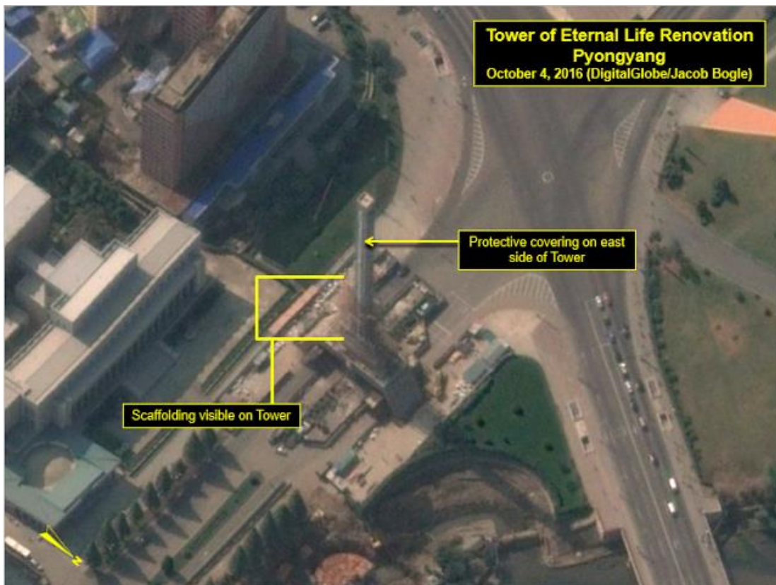
Figure 9: Scaffolding is visible on the Tower in this image dated October 4, 2016. (Image Credit: Google Earth/DigitalGlobe.)
