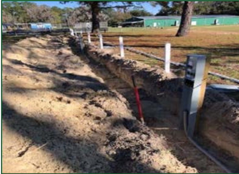
Power and water line installation
