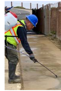
Applying concrete surface retarder
