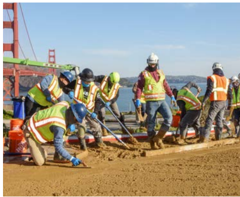
Placing & finishing pumped concrete
