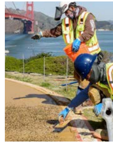
Placing/embedding special aggregate for later surface exposure
