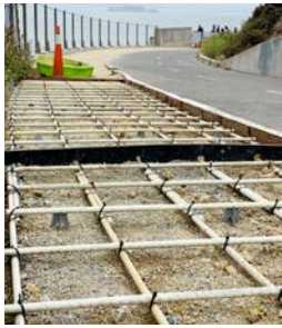
Site prep & glass fiber reinforcing bars installed
