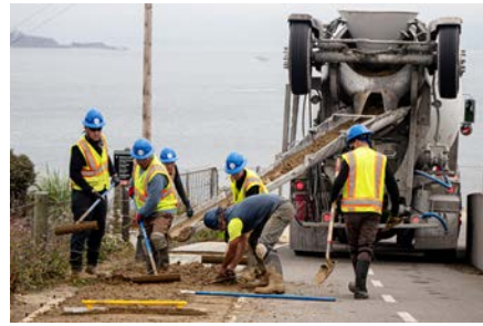
Placing truck discharged concrete
