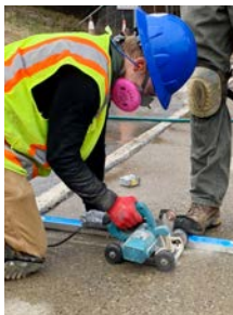
Saw cutting expansion joints on hardened concrete
