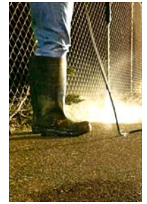
Night work to water blast & expose aggregate
