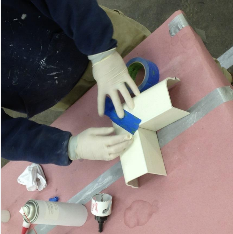
Tape outside of seam to prevent spillover
