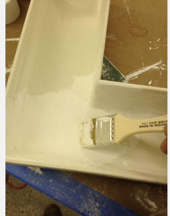
Use 2" Chip Brush or tongue depressor to wet out inside of seam with GutterGlue over fiberglass tape
