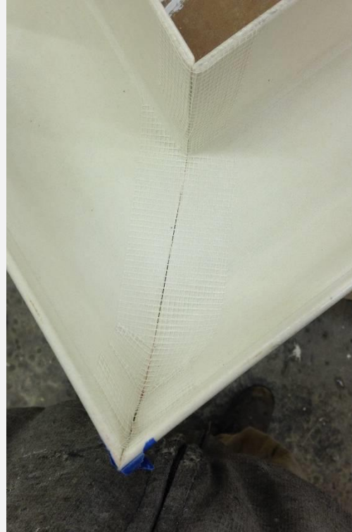
Lay FiberGutter Fiberglass Tape into joint. Cut tape to 10" pieces and stack 3 together for best results.
