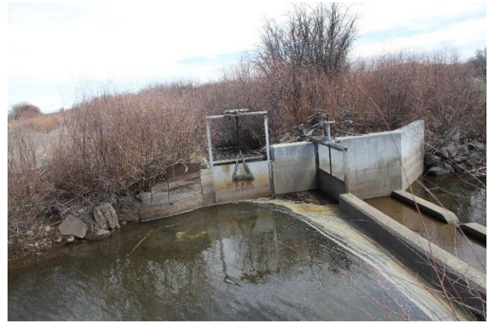
Headgate and diversion dam
