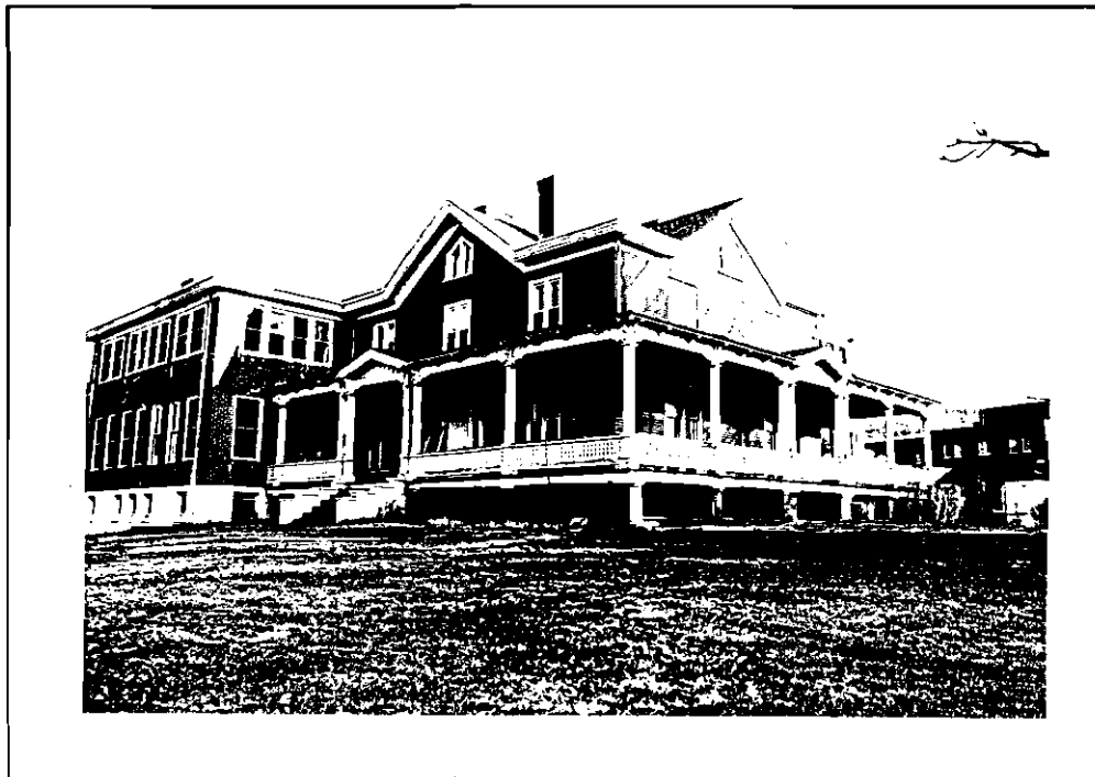
Figure 18. Blue Ridge Sanitarium (2-618).
