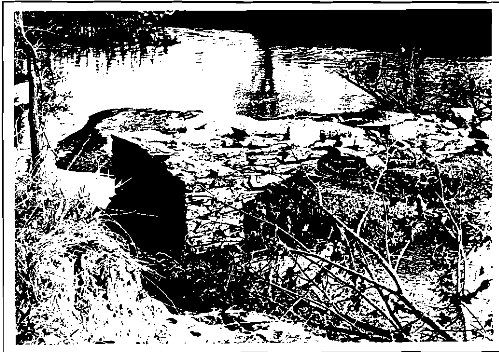
Figure 44. Stump Island Dam (2-1051).
