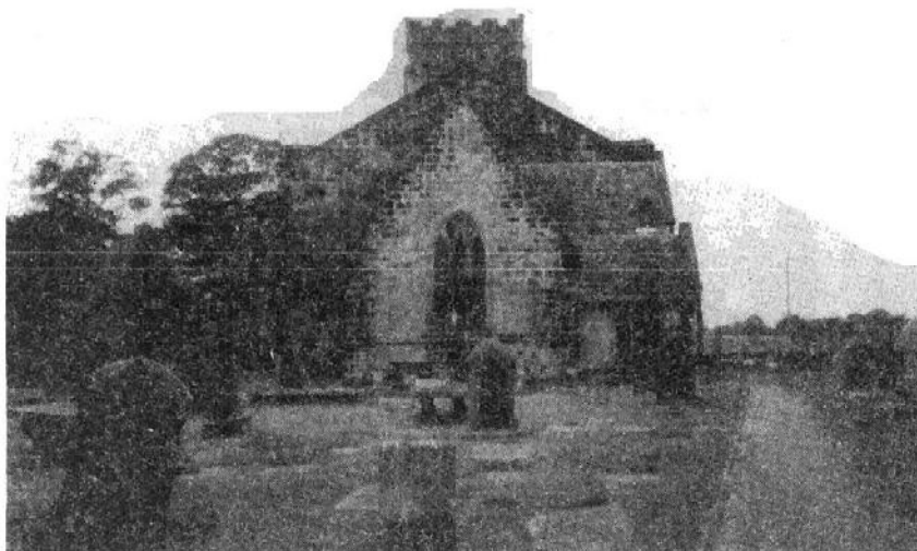
3. Medieval Chancel & East end of 1817 nave.
