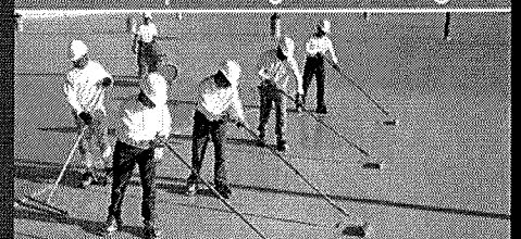
Building & Garage Restoration
