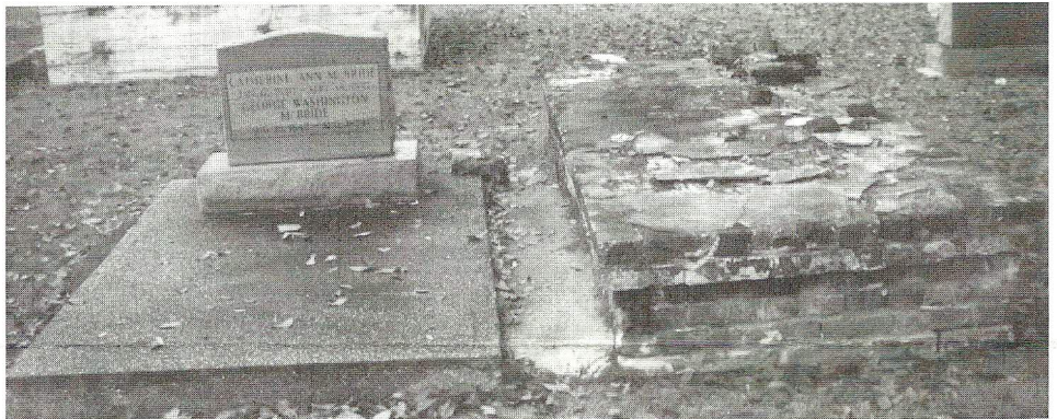
Adjoining Tombs, one in need of repair
