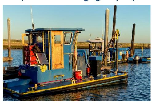
Underwater Earth Movers dredge works to complete the dredging of the boat basin at the Westport Marina. A total of 130,000 cubic yards was dredged from the boast basin.
