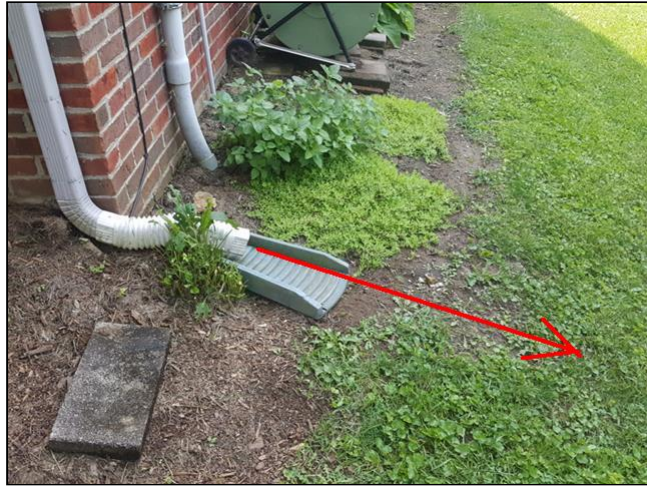
2.3 Item 6(Picture) rear right corner of home
