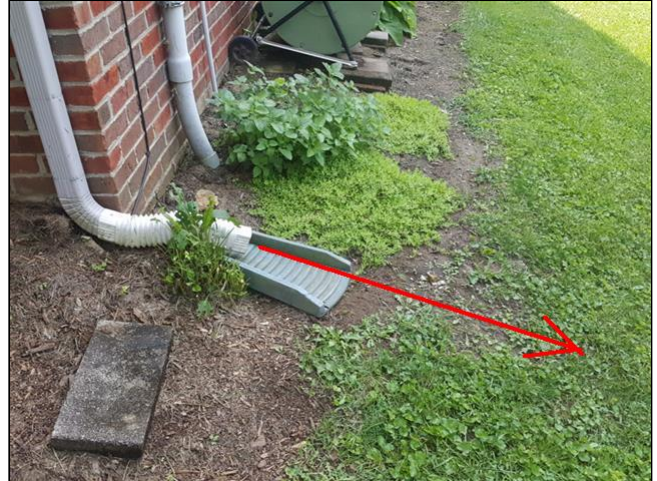
2.3 Item 6(Picture) rear right corner of home
