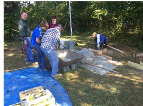
the gravel base. The other major project was to readjust the fire bricks in the ground along the edge of the back woods that are used for events such as water boiling during Field Day. The bricks were first removed from their places. Then the holes that held them were deepened and widened, then sand was added to provide a better foundation for the bricks. Finally the bricks were relaid in their original places.
