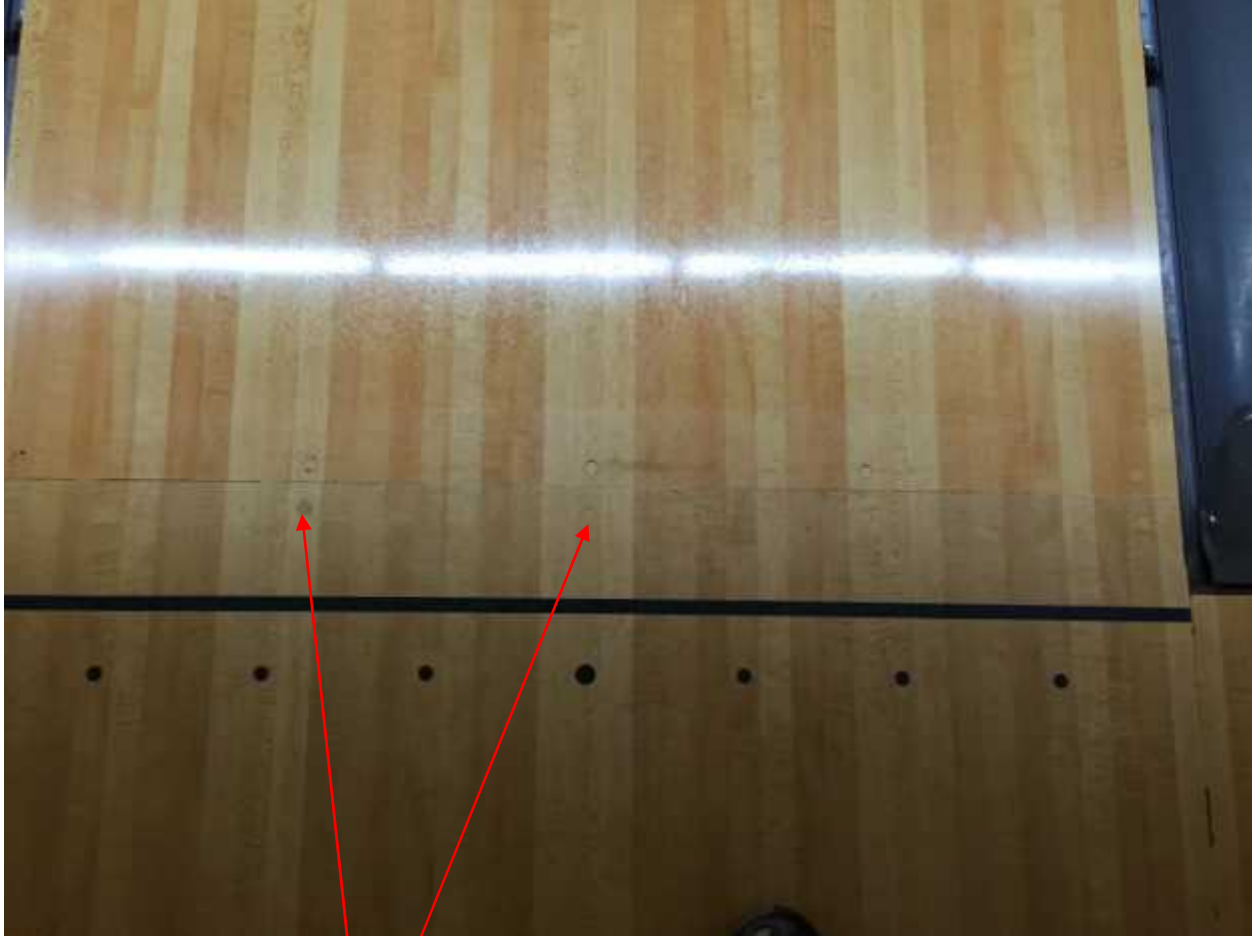
New Plunged Screwholes (5 on each end – 10 per lane) securing old panel.
