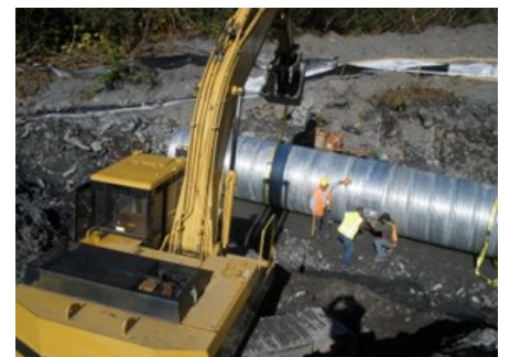
Mineral Creek Culvert Replacement
