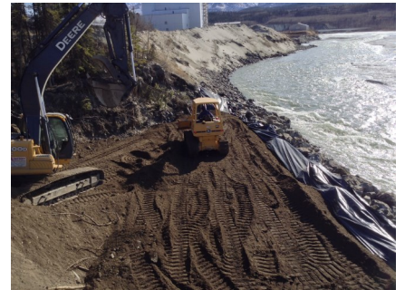
GVEA River Revetment
