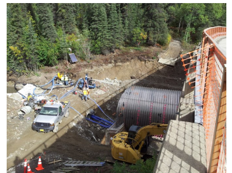
Rock Creek Multi-plate Construction
