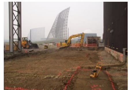
Clear AFB Bag House Upgrade Project
