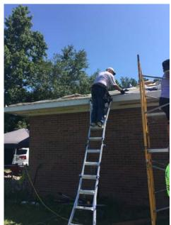
Chuck here, another day done. Today we had four kids and an adult from the other group from Winston NC. We got a late start, left the center at 8:15, and got to the jobsite around 8:45 and got the water damaged roof sheeting replaced, got the roof paper down, drip edge installed (except last 6 ft) waited most of the morn-
