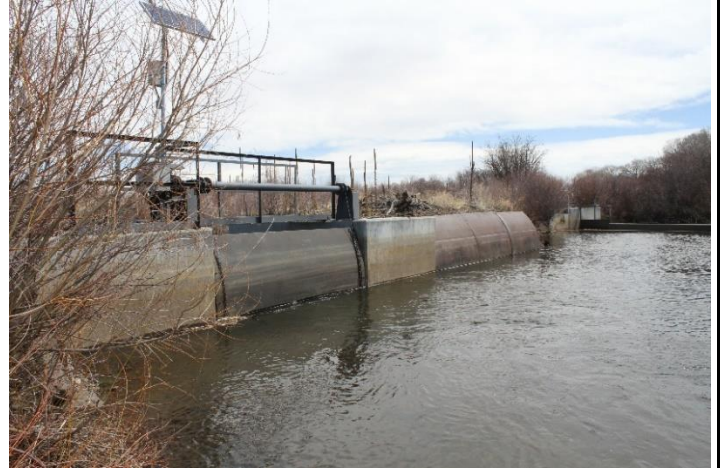
Headgate and diversion dam
