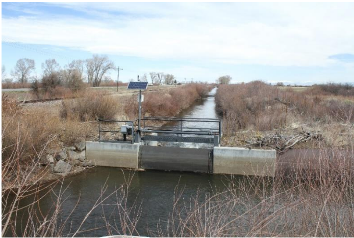
Headgate looking downstream
