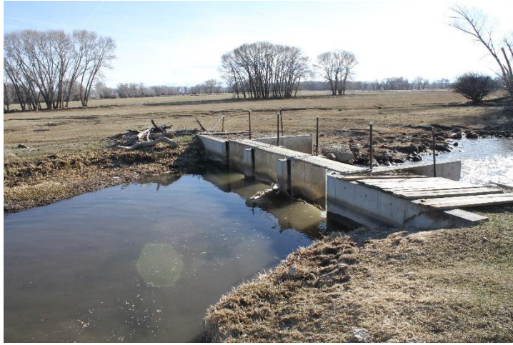
Weir looking downstream
