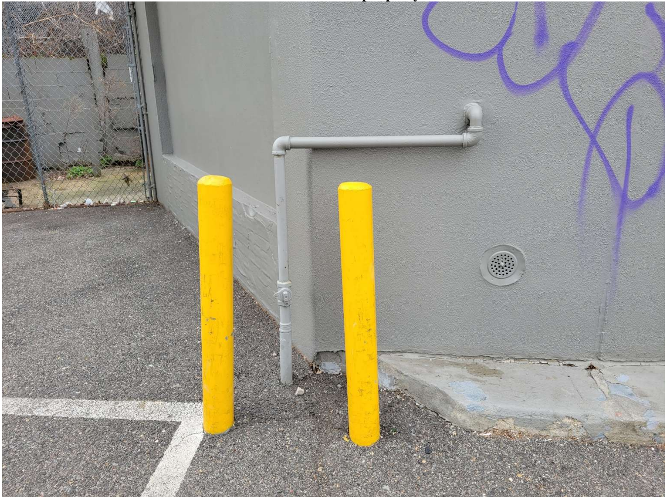
Gas Lines on the property
