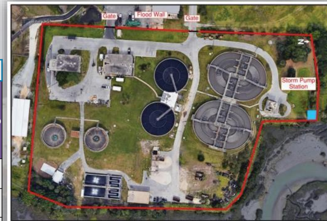
Figure 10: Perimeter Flood Wall and Pump Station
