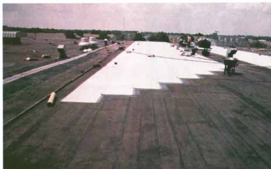
Staggering the end laps of cap sheets.
