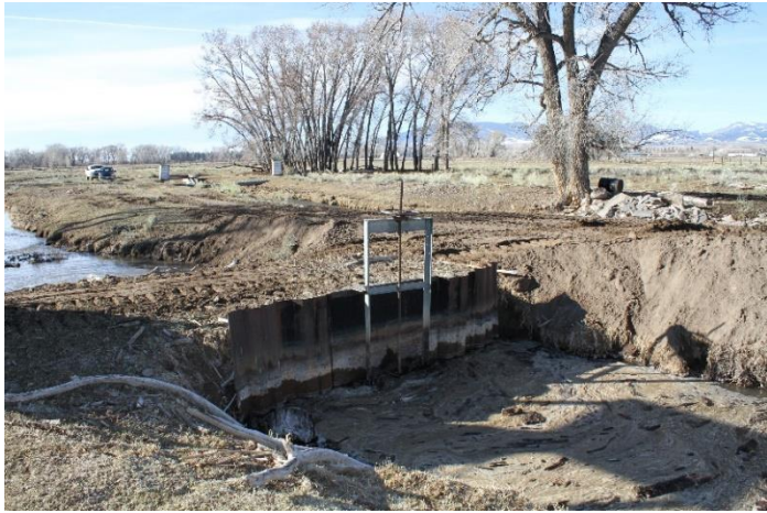
Headgate looking downstream
