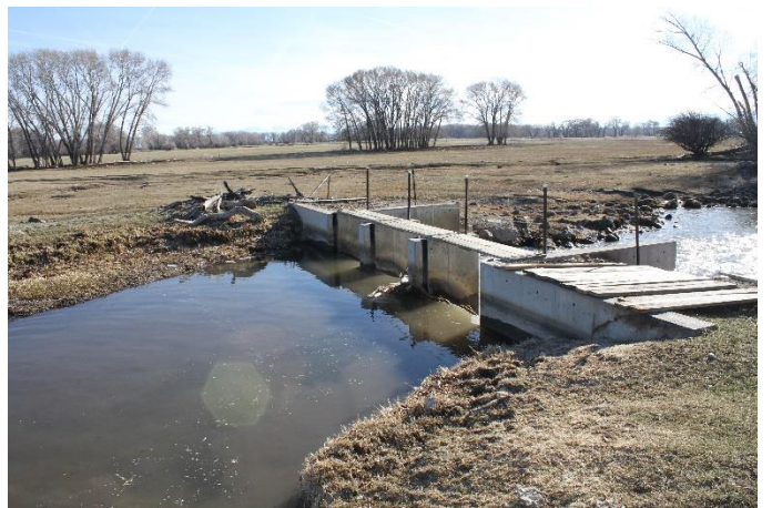
Feeder ditch diversion (Consolidated Slough Weir)
