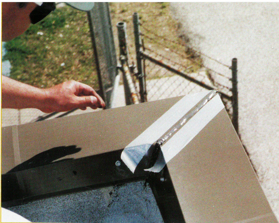
Installation of Band-aid joint with taped sides over seam in metal cap flashing.
