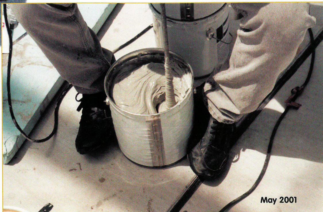
Right: Blending of a two-component sealant.
