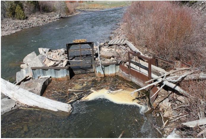
Headgate and overflow structure
