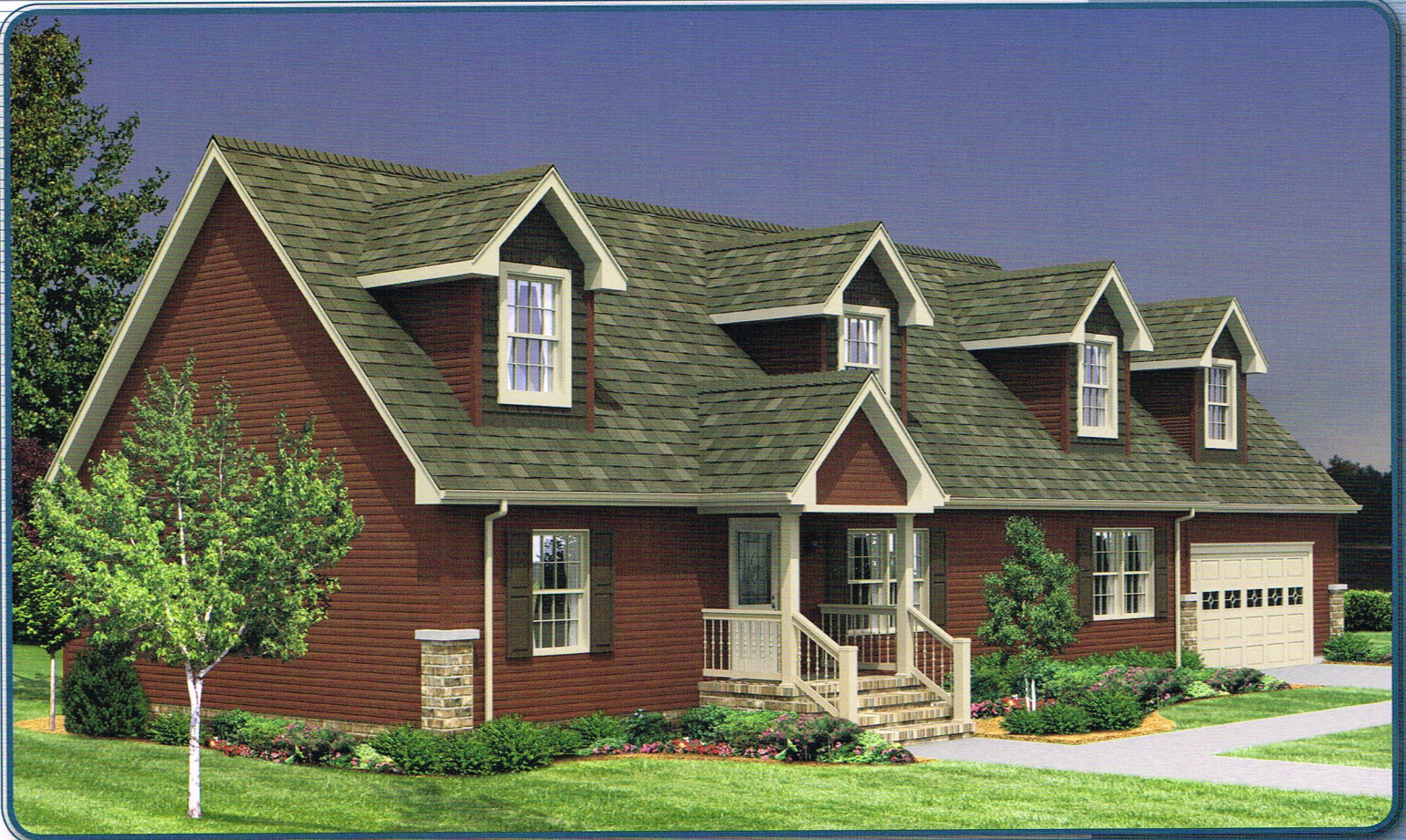
Some Exterior Features are Optional and Can be Built On-Site - Shown here with Optional Cape
