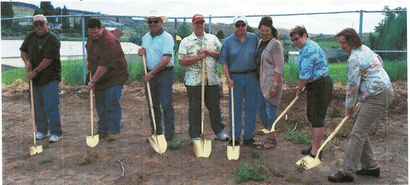
Ground Breaking Ceremony for Gronquist Building, May 3, 2016, pictured are members of the Columbia Hills Manor board, Gilliam County Court, and building Contractor (Pictured left to right) - Jeff Wilkins, Swaggart Brothers, Inc. project manager - Jim Hightower, Commissioner Mike Weimer, Mike Keown, Commissioner Dennis Gronquist, Tiah Devon, Alcenia Wright, Nancy Proctor.
