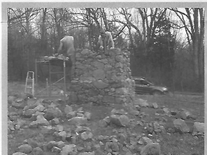
Chimney No. 1, restoration underway. Photo courtesy of Lynne G. Lewis.
