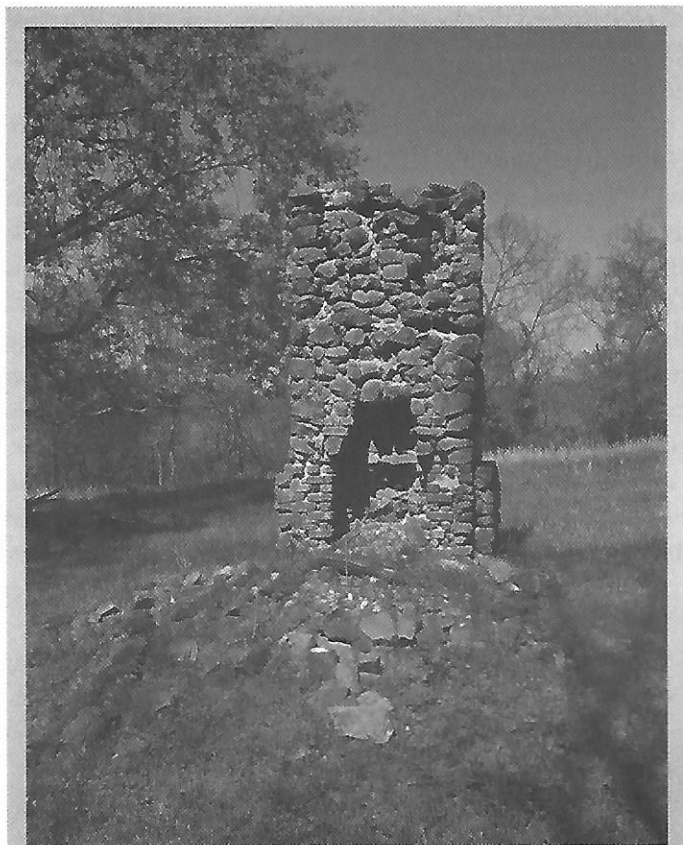
Chimney No. 4. This chimney was cleaned of overgrowth but did not need restoration. Note the method of creating the lintel. Photo courtesy of Bernice Walker.
