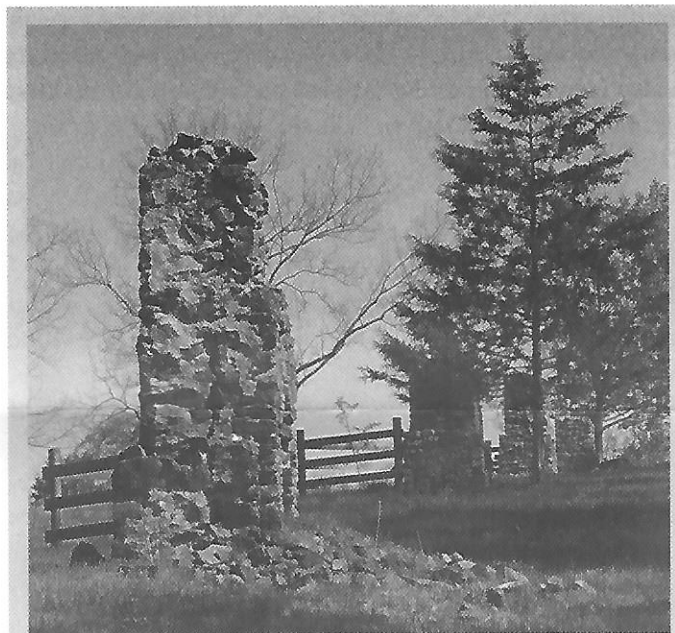
Chimneys 4 thru 1 (uphill), after restoration of 1-3 completed. Only chimney 5 cannot be seen. Photo courtesy of Bernice Walker.
