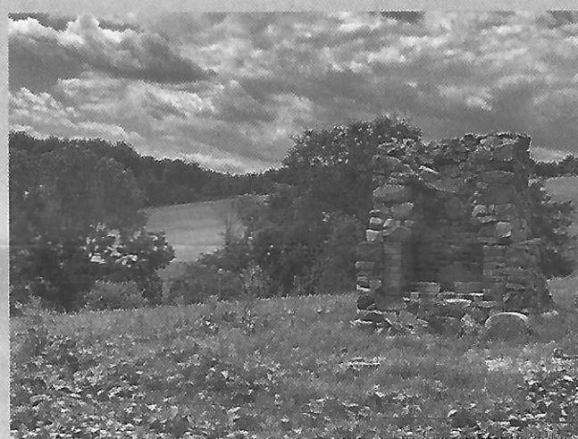
Chimney No. 1, after restoration was completed. Courtesy of Lyne Shackelford.
