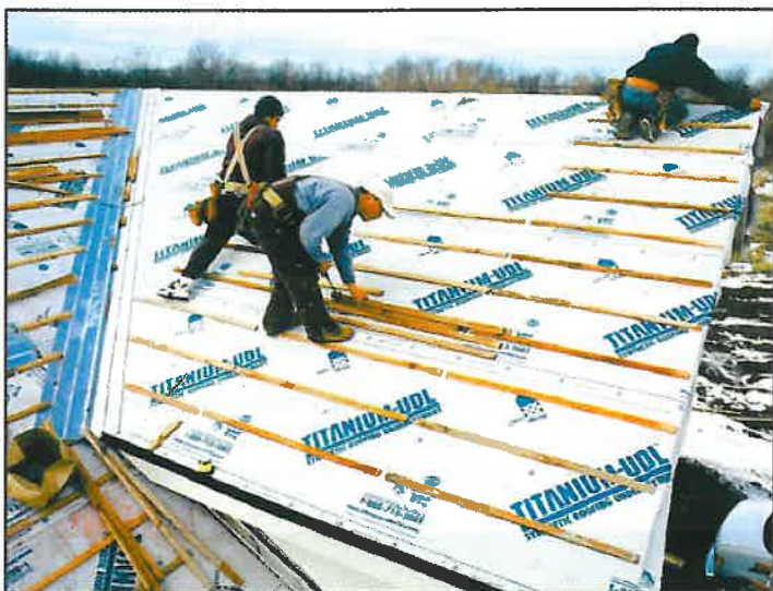
Typical synthetic underlayment installation under tile.
