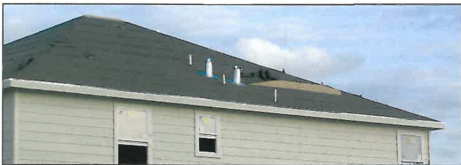
Felt underlayment displaced by wind.
