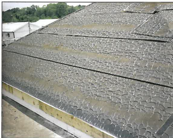
Wrinkled rubberized underlayment due to overexposure.
