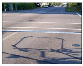
Figure 2. The Magnetic loop sensor placed at the road end before the junction.
