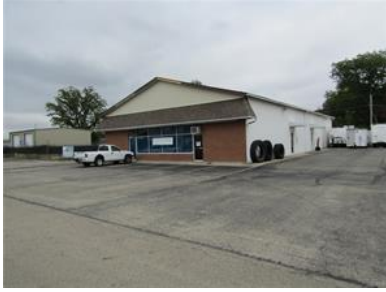
150 Industrial Drive Eaton OH 45320 2200
