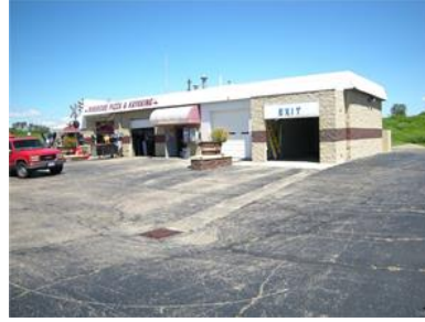
2401 Carmody Boulevard Middletown OH 45042 1705
