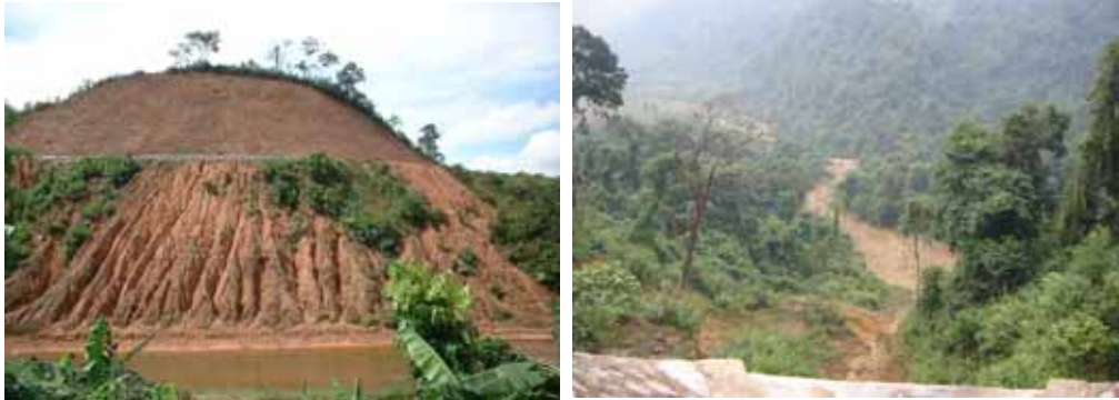
Photo 20: Left: Improper rock/soil waste disposal moves far downstream; right: impacting a village in A Luoi district, Thua Tien Hue province
