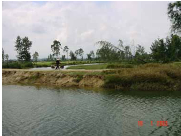
Photo 24: Vetiver, installed in a cross-hatched pattern, protects shrimp pond dikes in Quang Ngai
