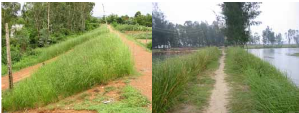
Photo 11: Left: Vetiver planted on river dike along Tra Bong River; right: lining the sides of an anti-salinity estuary dike along the same river
