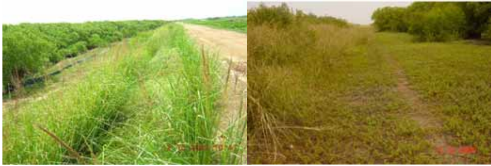
Photo 17: Planted behind natural mangrove on an acid sulphate soil sea dike in Go Cong province, Vetiver reduces surface erosion and fosters the re-establishment of local grasses.
