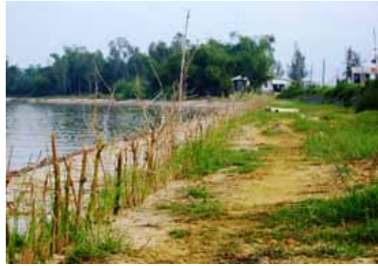
Photo 8: Left: March 2002: VS trial at the edge of a shrimp pond, where a canal drains flood water to Vinh Dien River; right: November 2002: mass planting combined with rock riprap to protect bank along Vinh Dien river
