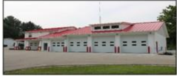
MFPD STATION 24 7606 E. State Road 45 Unionville, IN 47468
