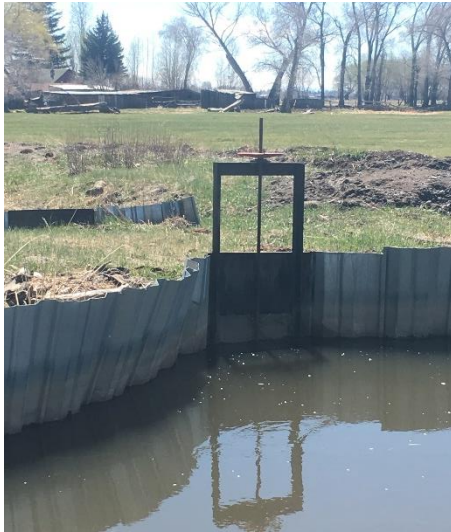
Headgate and return structure
