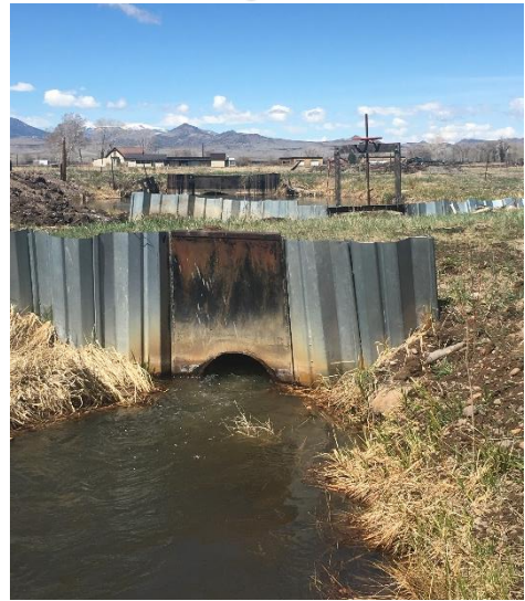
Headgate and return structure
