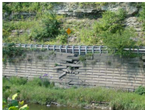
Route 8 Bypass Wall
