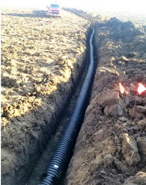
*Above: Tile being Installed for a series of 2 Sediment Basins in the Washington Lake Watershed*
