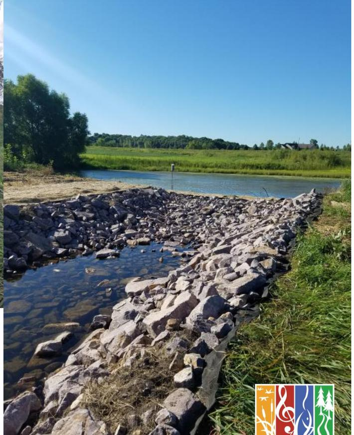
*Above: The before photo of the wetland outlet that was installed improperly years ago. The water had created a path under the concrete which drained the wetland from its original elevation. Right: Completed Project Rock Lined Outlet Control Structure Which Restored a Wetland near Montgomery*
