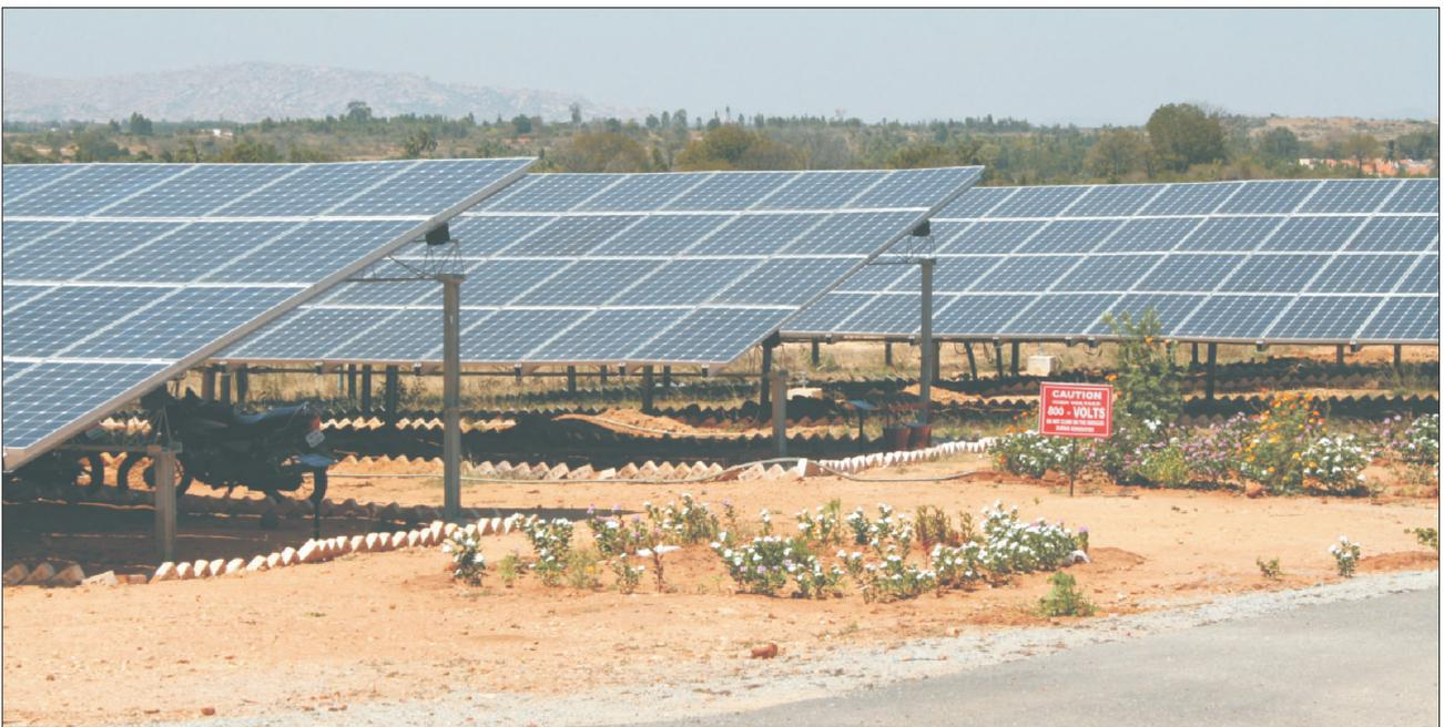
Figure 19: Photo of PV Plant showing the modules mounting structures inclined at 15°.
