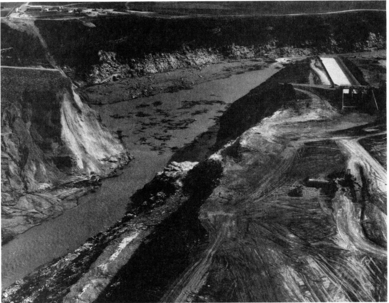
Figure 5-1. The Teton Dam, a Bureau of Reclamation project, collapsed in 1976 killing 11 people and causing millions of dollars in damages. The dam's collapse illustrated, once again, that structural solutions to flood problems are not without inherent risks.
