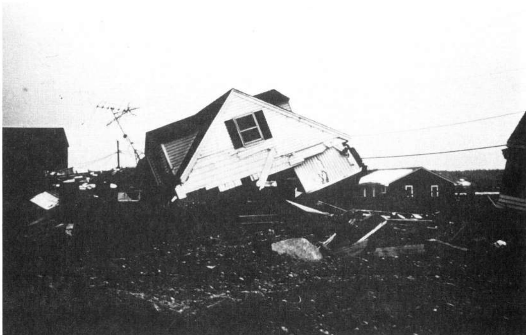
Figure 6-6: Buildings in the path of coastal floods seldom just get wet. Erosion worsens flooding as well as causing physical damage. Source: Jon Kusler.
