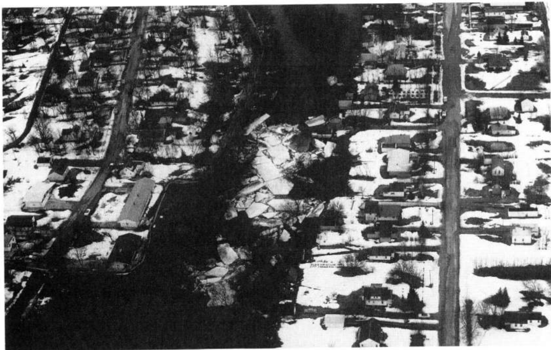
Figure 10-3. Large chunks of ice have jammed at a small dam. Source: St. Paul District, U.S. Army Corps of Engineers.
