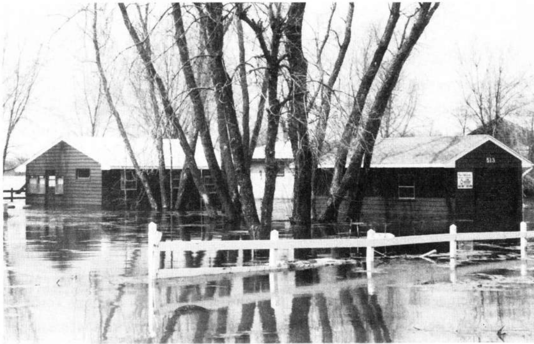
Figure 8-1. When these photos were taken, these homes on Lake Pulaski, Minnesota had been under water for approximately three years. See discussion in Appendix 8-A. Source: Minnesota Dept. of Natural Resources.
