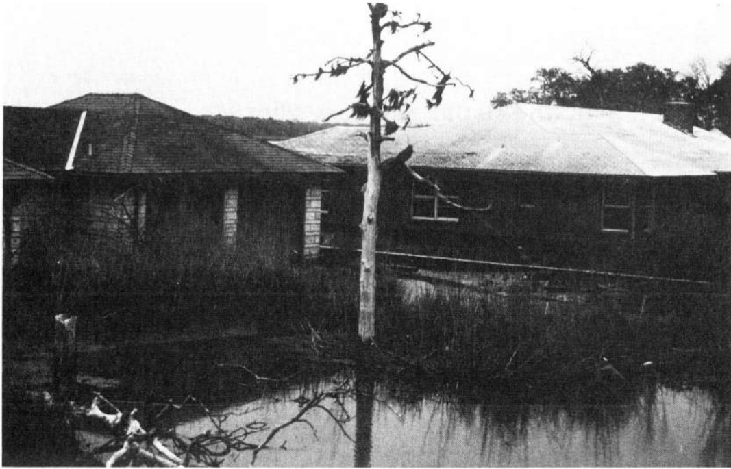
Figure 9-1. These houses in Brownwood Subdivision are flooded by daily tides because withdrawal of fluids has resulted in 2.5 meters of subsidence. Source: R. Platt.
