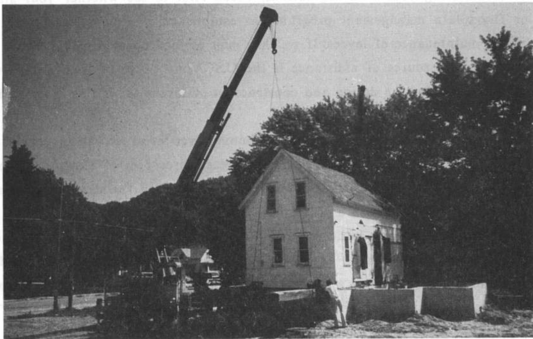
Figure 4-3. House behind levee in Soldier's Grove, Wisconsin being elevated after severe flooding in 1978. Source: T. Hirsch.
