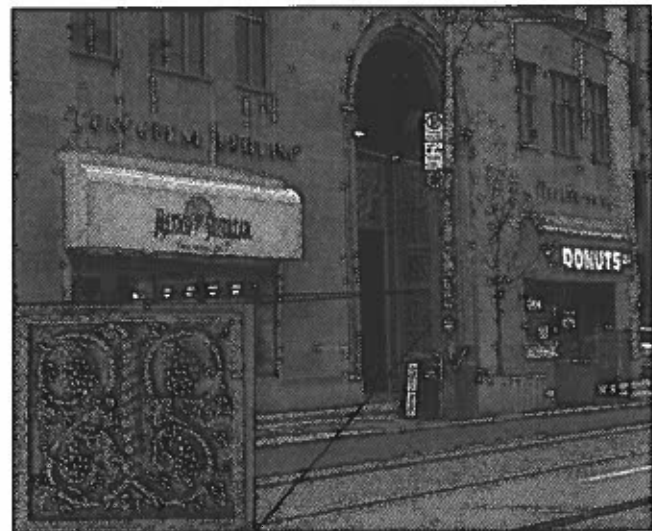
The Concourse Building on Adelaide Street in Toronto with an example of the elaborate stonework shown (inset).
