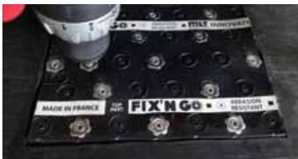
Secure bottom of the **Fix'N Go** by installing all the screws alternating sides and rows.
