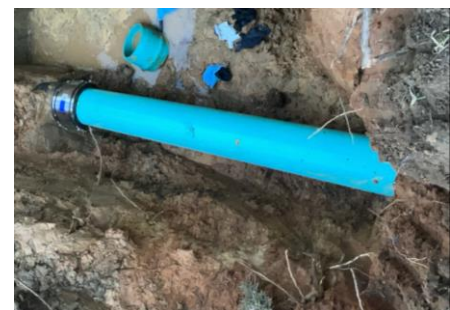
Forest MCWI Sewer Improvements
