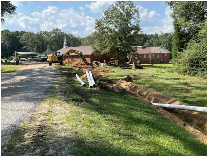
Polkville DRA Water Improvements
