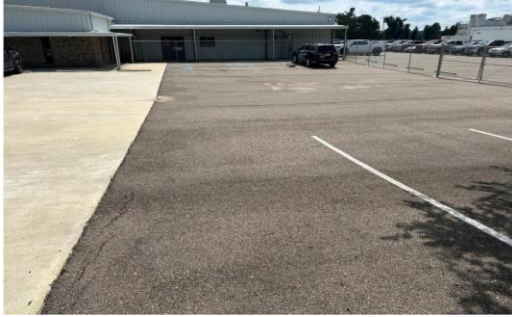
Jasper County DIP Hol-Mac Parking Lot Improvements
