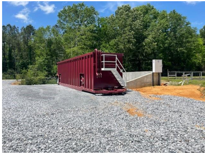
Lake CDBG PF New Wastewater Treatment Plant
