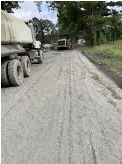
Leake County CDBG PF Road Improvements
