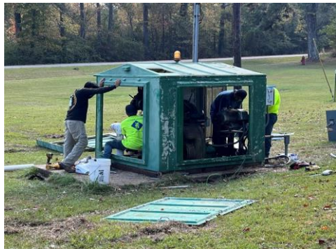
Heidelberg MCWI Wastewater Improvements
