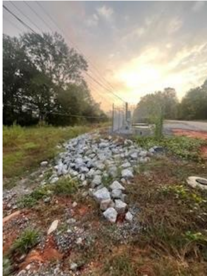
Marion MCWI Sewer Lines
